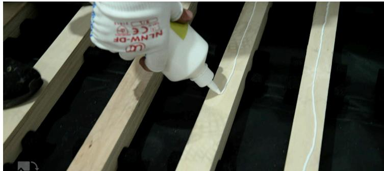
5. Apply P300 adhesive to top of flexjoists and lay 18mm T&G plywood with all T&G joints glued using P300 PVA adhesive.
