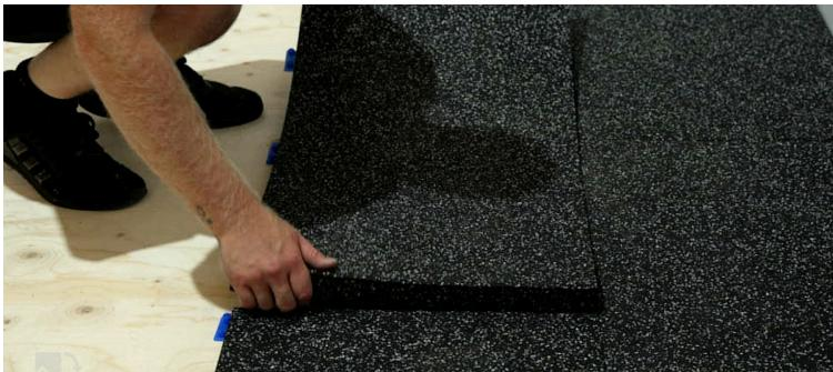
9. Lay Gymflex 40mm tiles with clips, lay in a brickbond pattern with fixing clips on reverse side. Use a rubber mallet to ensure fixings are correctly located and floor is sitting flat. Leave 10mm expansion to all abutments.
