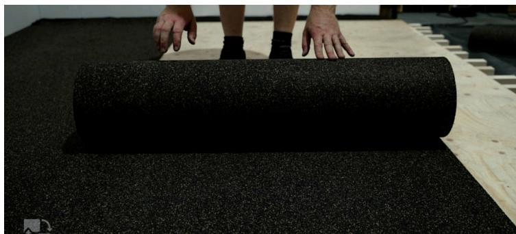
7. Lay 5mm Shockroll on plywood, joints taped using Gymflex Shock tape.
