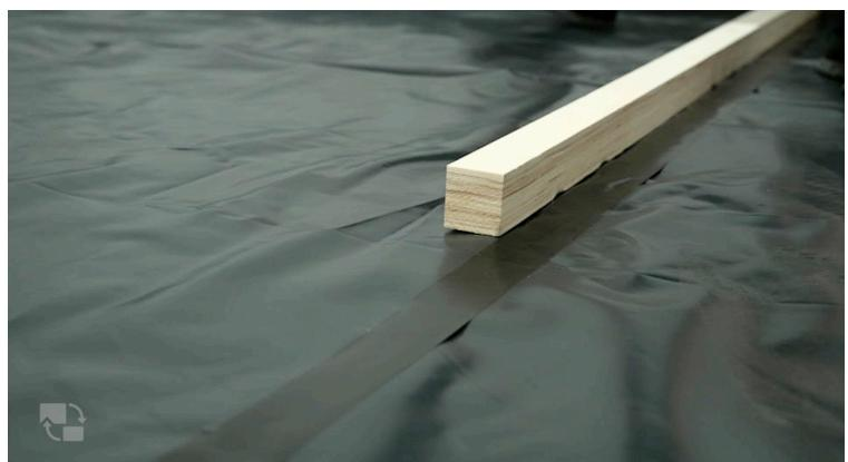
2. Flexjoist Centres to be set out at 150mm and cradles along the flexjoist at 300mm.
