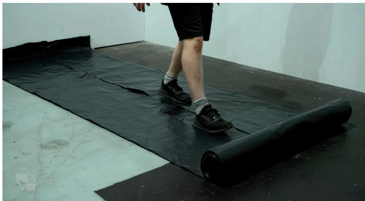
1. Lay 1000 gauge polythene with 150mm overlapped and taped joints. Lap up wall passed finished floor height.
