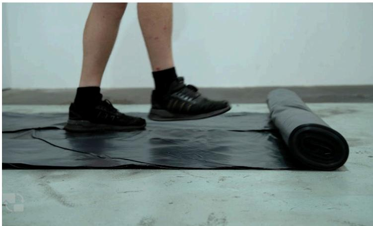
1. Lay 1000 gauge polythene with 150mm overlapped and taped joints. Lap up wall passed finished floor height.
