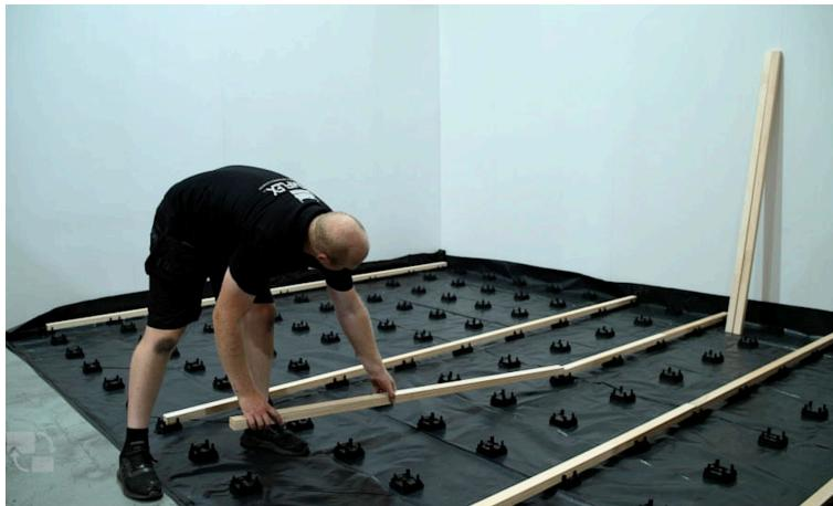
4. Fit Flexjoist to cradles, ensuring each row is staggered to make sure floor is fully tied in. Leave minimum of 40mm expansion off wall on ends of every Flexjoist.
