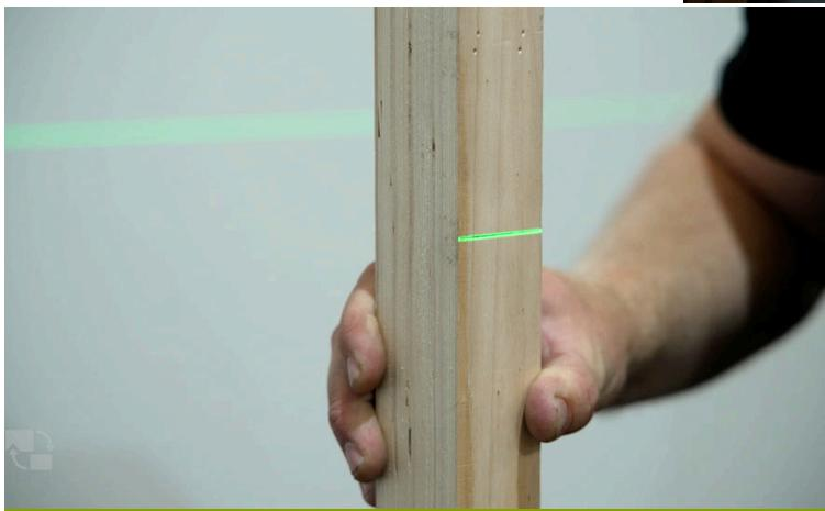
3. Sports cradles to be adjusted to datum using Laser level and New Era packers fitted to cradles.
