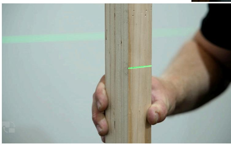
3. Sports cradles to be adjusted to datum using Laser level and New Era packers fitted to cradles.
